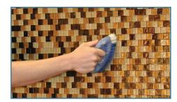
**Step 9** After a full 24 hours (some installations may require extended cure times) use water and a nylon scrub-brush to remove residual glue from the tile. Clean rinse and towel dry.
