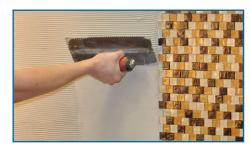
**Step 3** Use the flat side of the trowel to flatten the notches and achieve a smooth, consistent thin-set setting bed.
