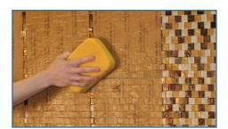
**Step 6** After 15-30 minutes, (floors can be removed sooner) lightly wet the paper. Keep the paper wet by wiping with a damp sponge several times over a 5-10 minute period. After the paper has absorbed the water, the glue will release.
