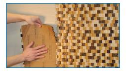
**Step 4** Apply mosaic sheets to the thin-set setting bed, paper side towards you, with light, even pressure. Periodically, check thin-set for skinning (slight drying). If skinning occurs, remove thin-set and reapply.
