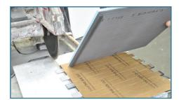
Step 4 With the saw turned off, place the mosaic sheet, paper side up, on the cement board covered saw tray and align the cut.
