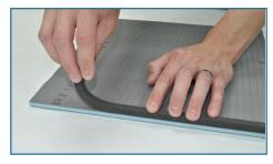
Step 3 Cut another piece of 1/4" cement board to a square size that is larger than a sheet of mosaics. Apply a strip of self-adhesive, compressible, foam weather-strip to one edge of the cement board.
