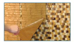
**Step 7** Peel the paper from the tile starting at the corner. Removing the paper while the setting material is still fresh allows for individual tile adjustment and re-inspection of color consistency.
