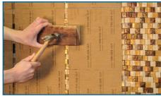
**Step 5** To achieve the flattest possible surface, lightly tap the sheets with a wooden beating block and a finish hammer. To unify sheet transitions, tap from one sheet to the next.
