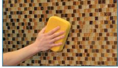
**Step 11** Allow grout to set-up (firm) and smooth finish with a damp sponge. After approximately 2 hours remove grout haze with a lightly damp sponge.
