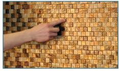
**Step 8** Straighten individual mosaic tiles prior to final set with the goal of creating a consistent overall field of mosaics. To eliminate the sheet pattern, pay particular attention to the transitions between sheets.
