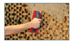
**Step 10** Apply grout with a rubber grout float, forcing grout into joints until full.
