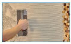
**Step 2** To establish the proper depth of the setting bed, use a 3/16"x1/4" v-notch trowel to apply additional thin-set and comb full notches in one direction.
