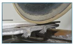
Step 2 Adjust the blade height so the blade cuts through 1/2 of the cement board thickness.
